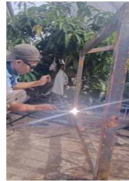
(c). Penyambungan besi siku
